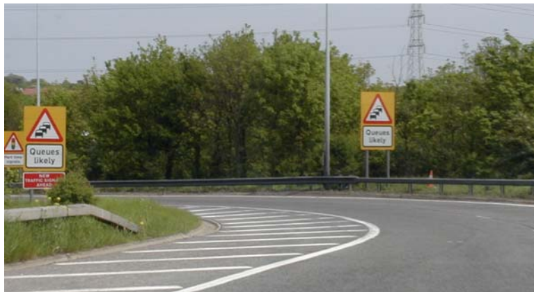
Typical advanced fixed signs
