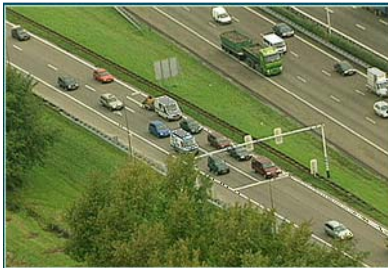
Birds eye view of two-lane ramp meter
